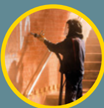
Low-pressure blasting
